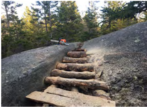
Log steps lead to a section of open granite ledges on the new Vinal Cove Trail. Stewardship and photo by Kerry Hardy.
