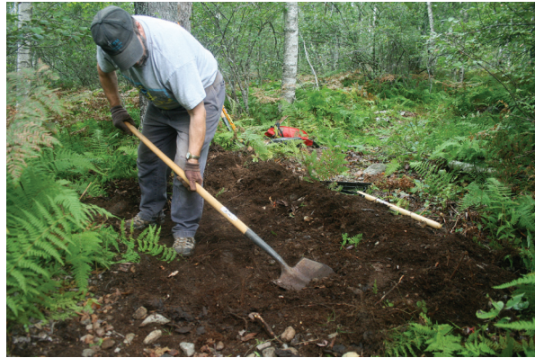
VLT volunteer Rick Morgan finishing work on a waterbar to control erosion on the trail to Fox Rocks. Photo by Kerry Hardy.
